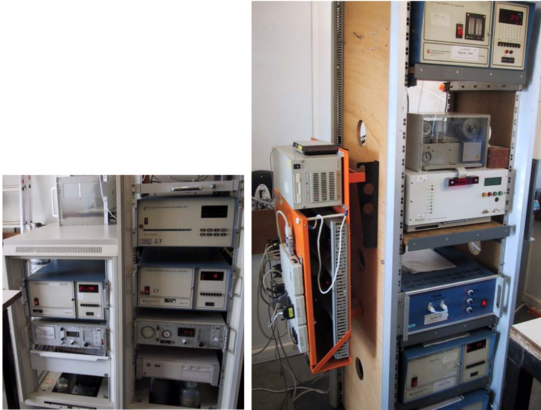
Figures 1a and 1b: Measurement equipment set up in the station; Left the LUEN monitors and right those of RIVM.
